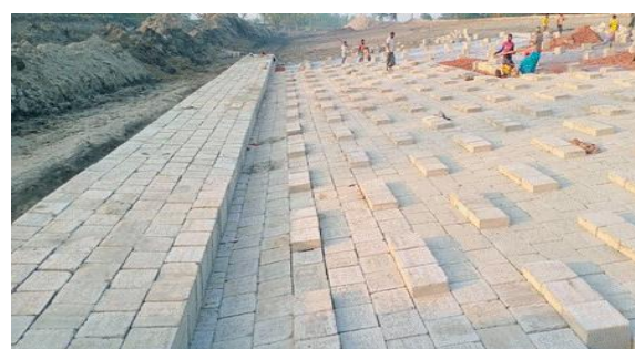
Figure 3-27: Ongoing Slope Protection Works (Polder 40/2), Barguna
