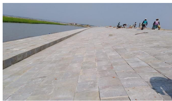
Figure 3-10: Completed Slope Protection Works in Polder-32
