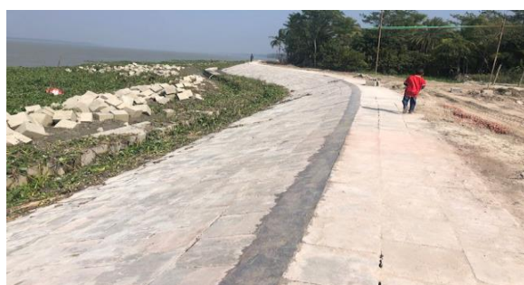
Figure 3-26: Bank Protection with Pitching Works (Polder 39/2C)
